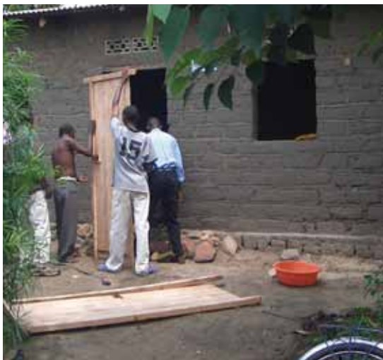
Here our volunteers are attaching a door to a new home.
