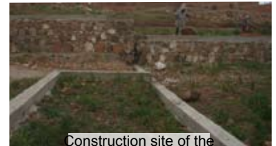
Construction site of the orphanage & school
